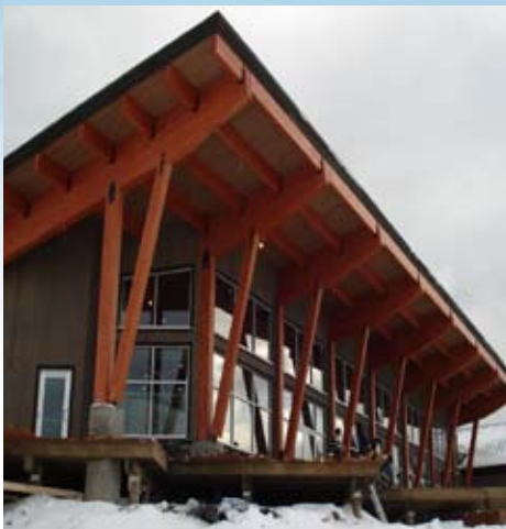
THE DAY LODGE ADDITION IS SHAPING UP NICELY. PHOTO: APRIL NORTH
