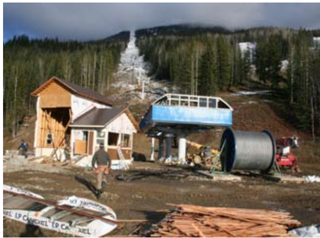
WORKERS PREPARE TO SPLICE "THE REVELATION" GONDOLA WIRE. PHOTO: BILL BLACK.
